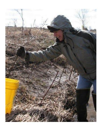
Example of Live Stake Streambank Being Installed.
